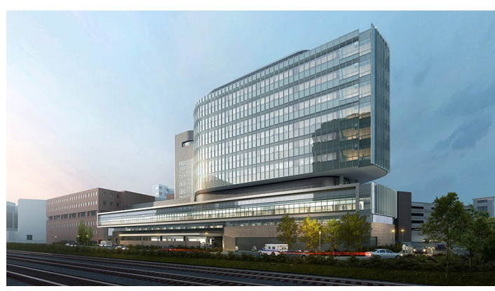
Tackling the hospital shortage with modular construction
